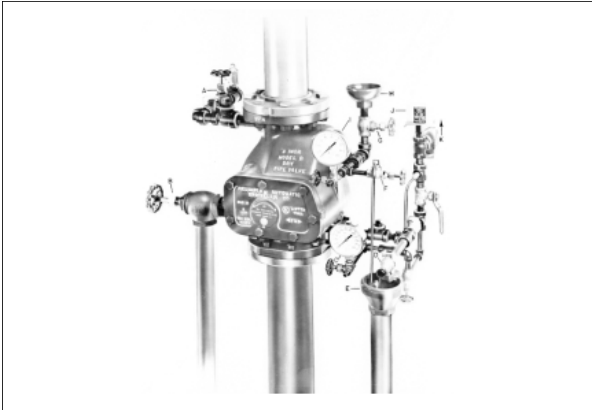
Fig. 76. Trim on Reliable Model D dry-pipe valve
