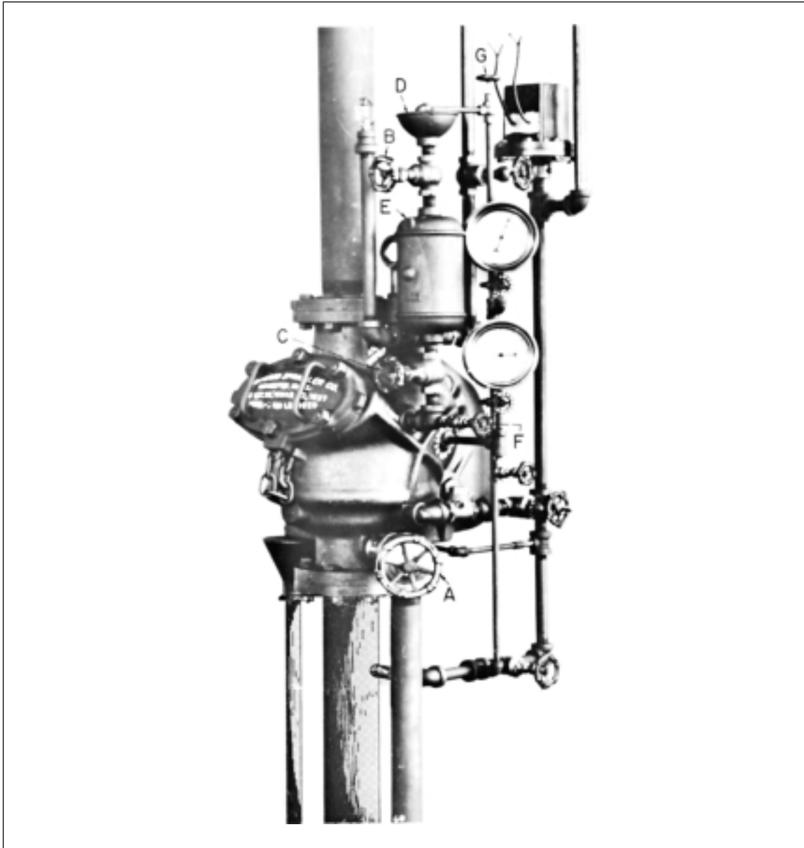
Fig. 82. Rockwood dry-pipe valve trim.
