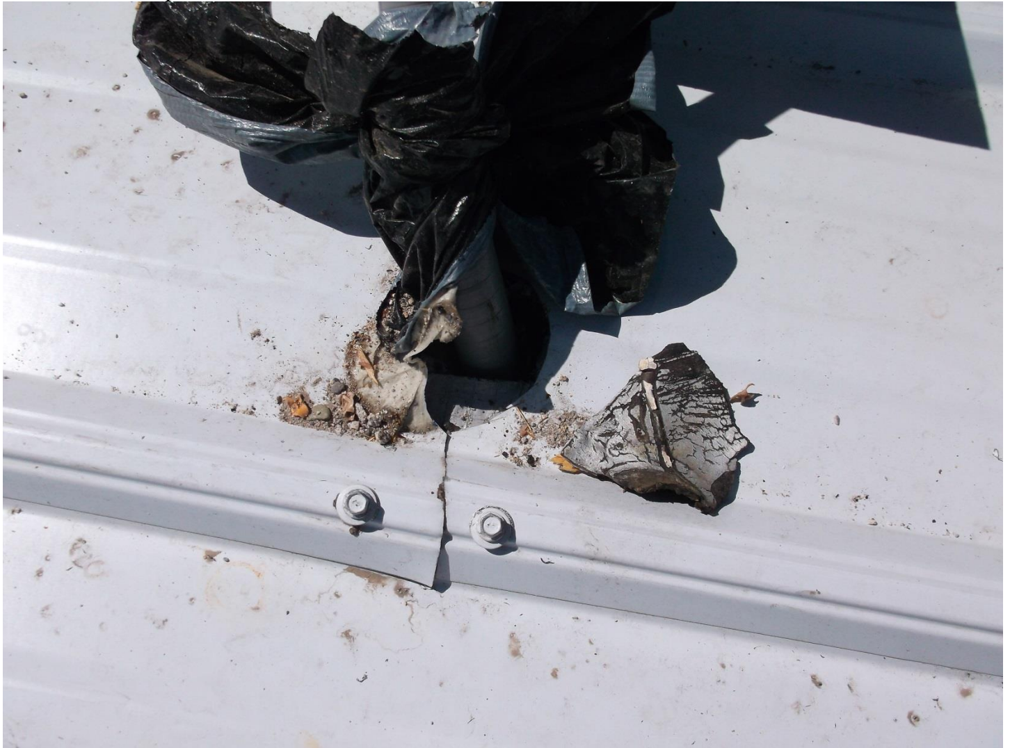
Electrical conduit penetration thru roof
