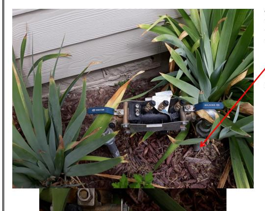
The lawn sprinkler Zurn-Wilkins model 375 RP, "appears" to be supplied via a tap-off from the fire suppression riser stack.
