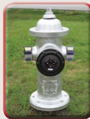
Hydrant Secured with (2) Knox SecureCaps and (1) Knox StorzGuard
